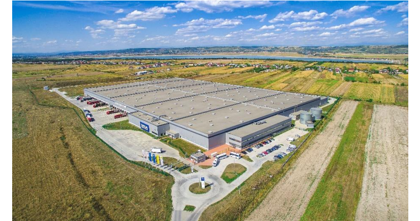
Facility in Piteşti
