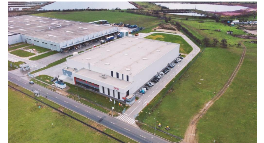
Facility in Oradea
