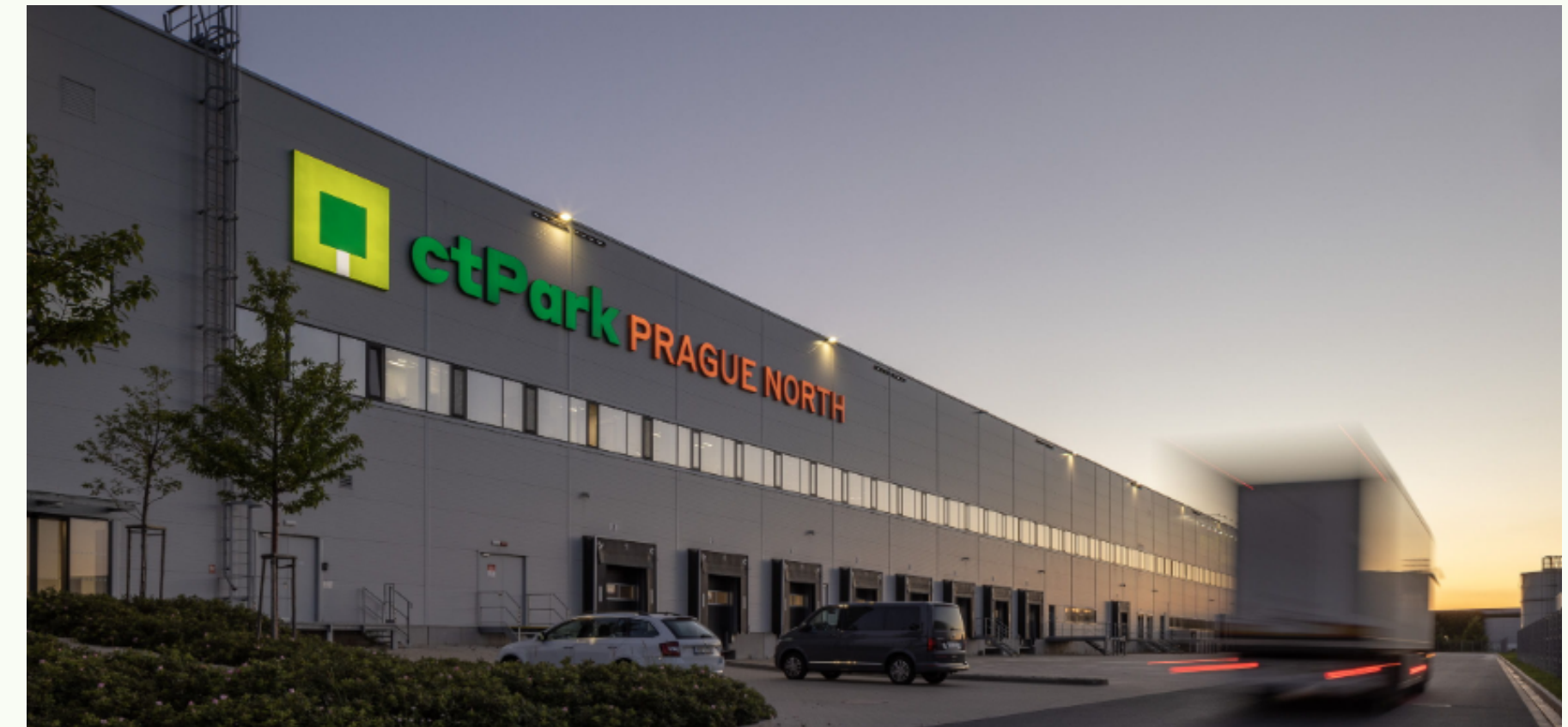
Most sustainable logistic park in Czech: CTPark Prague North
